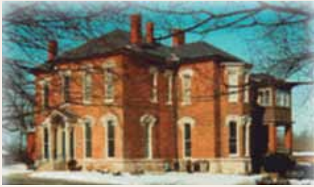
The Elmhurst Community Building (provided by the The Community Foundation of Greater Lafayette)
